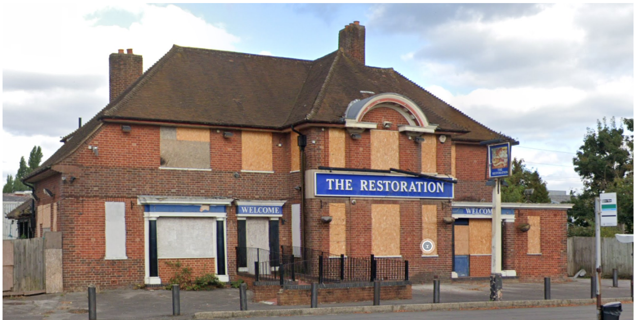
View of the Restoration Public House in 2021, Google Streetview
