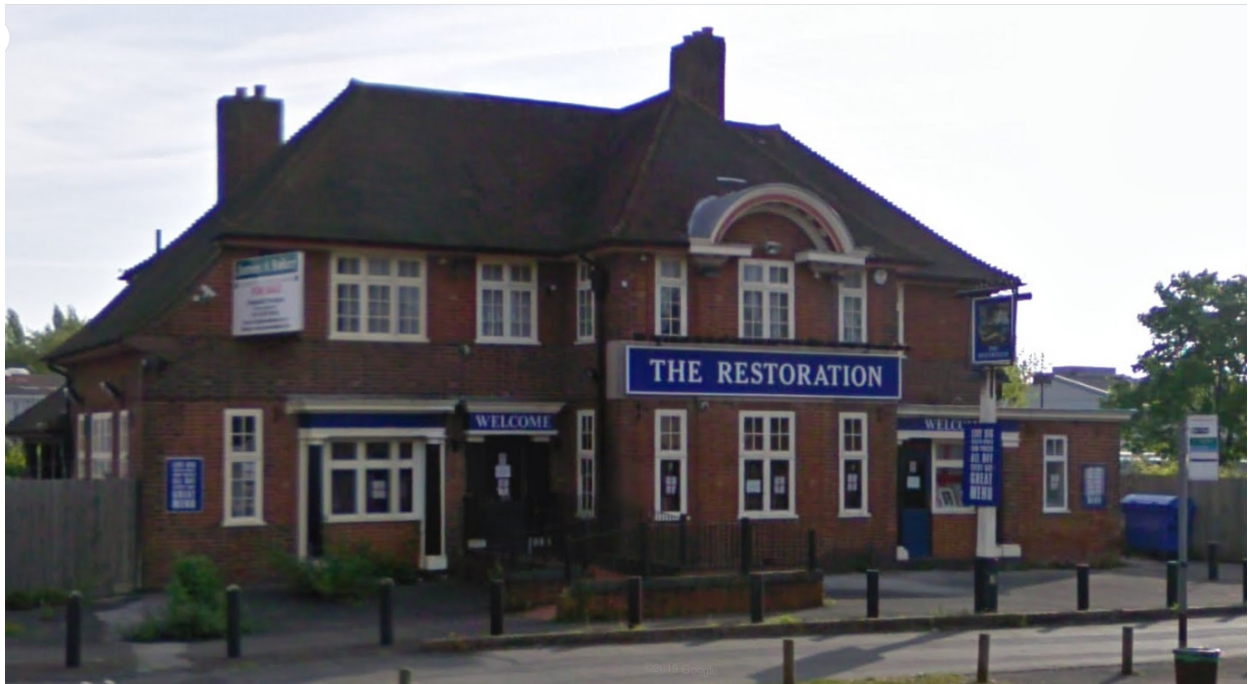
View of the Restoration Public House in 2009, Google Streetview
